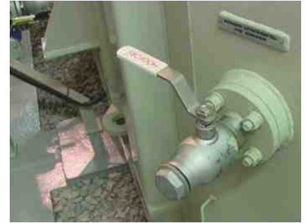
Figure 8. Recommended installation locations for the moisture sensor. The oil cooling circulation line (left) is the ideal location for measurement in both forced and free circulation cooling implementations; installation through outer wall of transformer tank (right).
