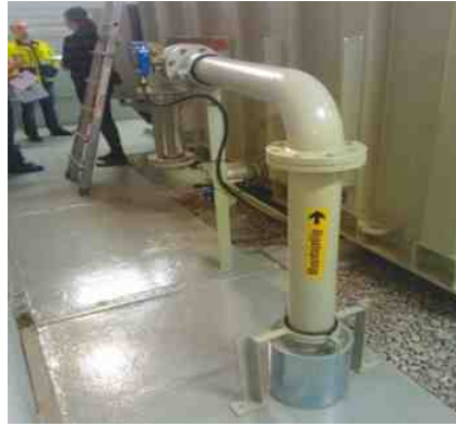
Figure 8. Recommended installation locations for the moisture sensor. The oil cooling circulation line (left) is the ideal location for measurement in both forced and free circulation cooling implementations; installation through outer wall of transformer tank (right).
