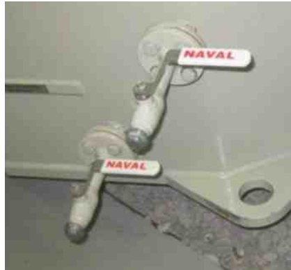
Figure 9. Non-recommended installation locations for the moisture sensor. Oil sample connector near the bottom of the transformer tank (left); expansion tank (right).
